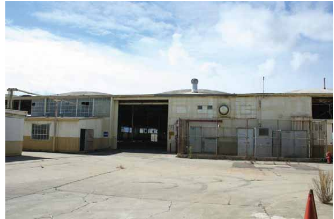
Building 156 - Warehouse, East Elevation, San Diego, California, October 2009.
