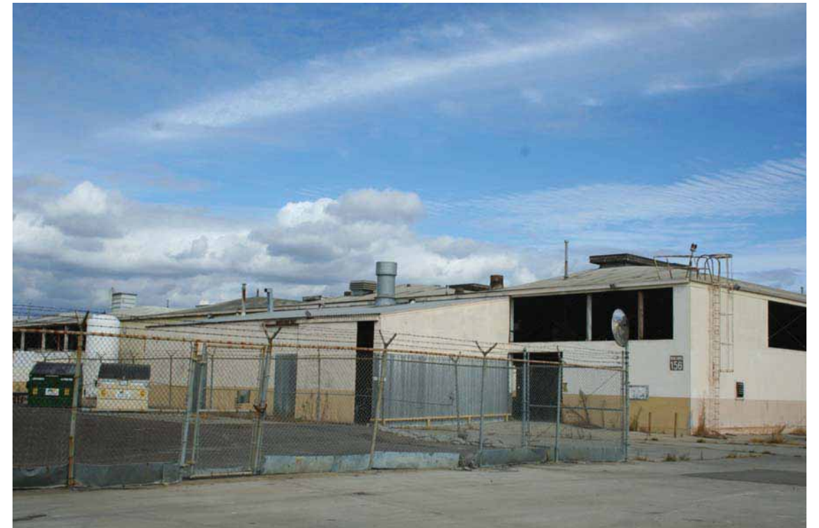
Building 156 – Warehouse, West Elevation, San Diego, California, October 2009.
