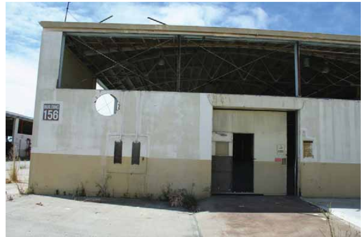
Building 156 - Warehouse, south corner of East Elevation, San Diego, California, October 2009.
