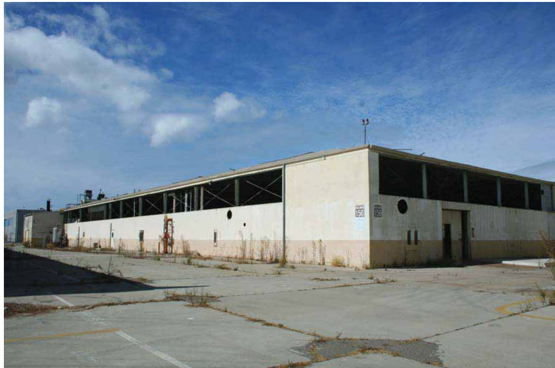
Building 156 – Warehouse, Northeast Oblique, San Diego, California, October 2009.
