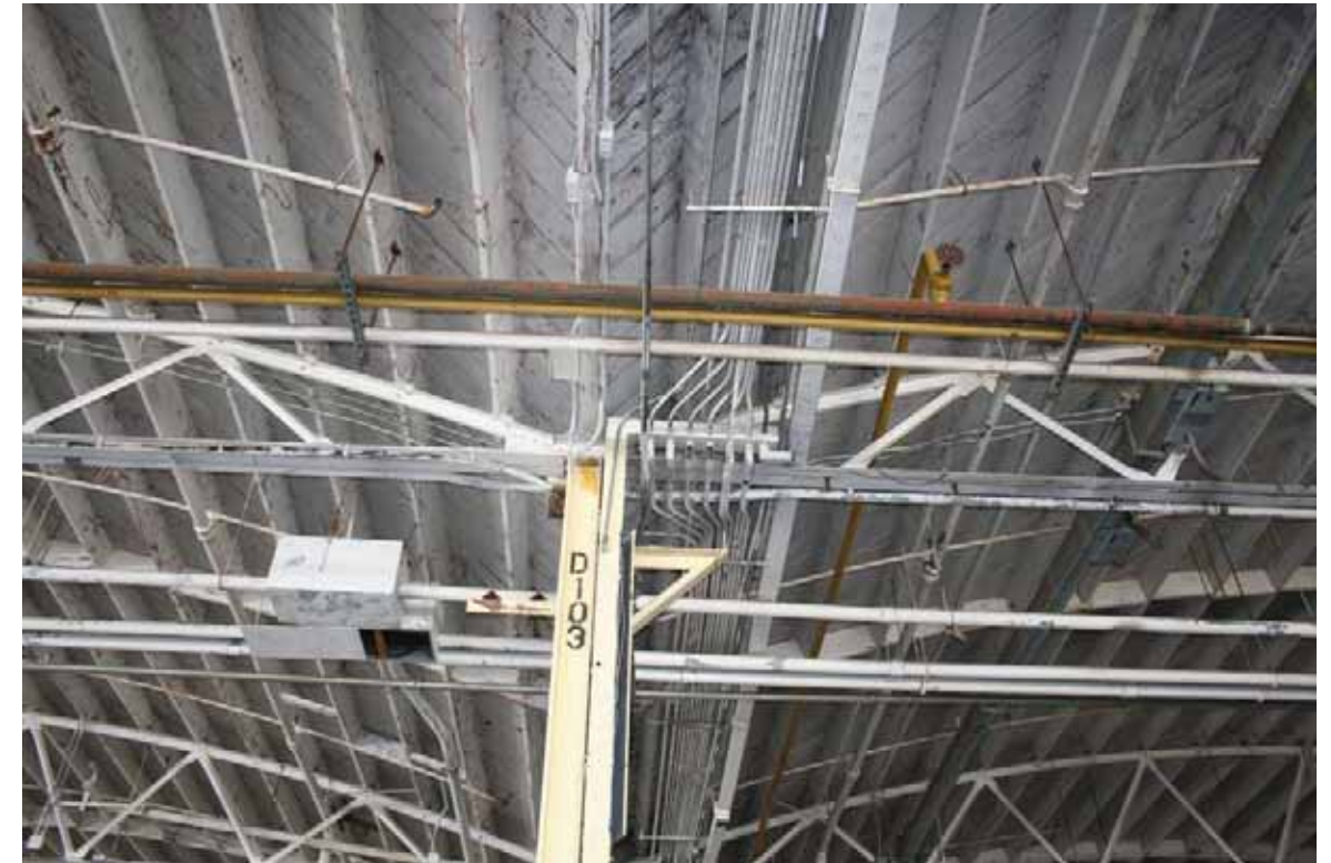
Building 156 – Warehouse Interior, ceiling detail, San Diego, California, October 2009.
