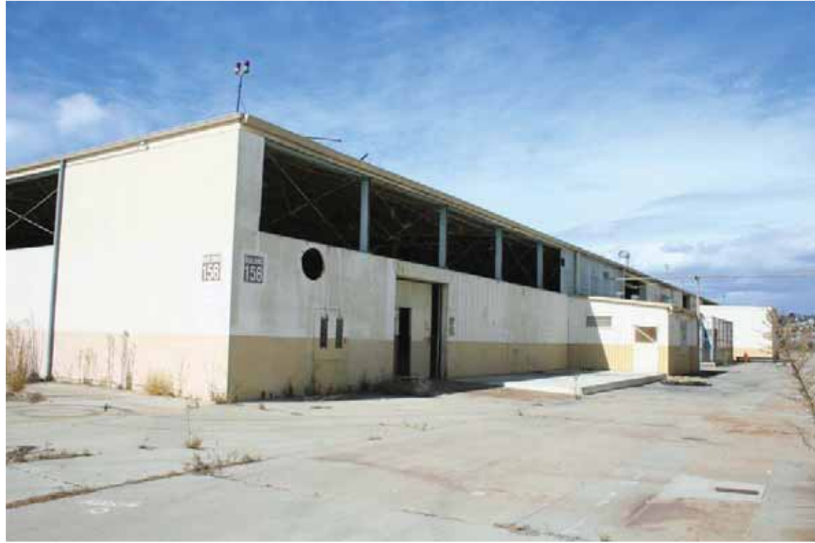
Building 156 – Warehouse, East Elevation, facing Northwest, San Diego, California, October 2009.
