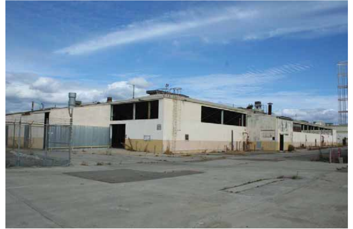
Building 156 – Warehouse, Northeast Oblique, addition on South Elevation, San Diego, California, October 2009.
