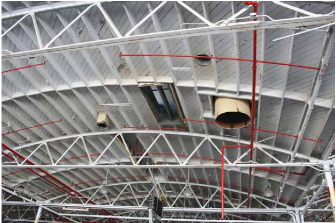
Building 152 – Jet Engine Drone Assembly Building Interior, ceiling detail with the opening for the roof monitor, San Diego, California, October 2009.
