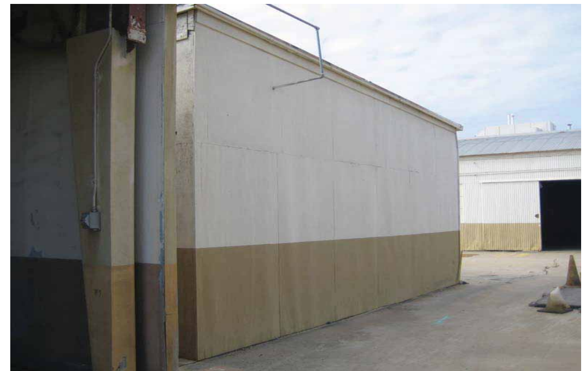
Building 129 - Sandblasting Shed, Northeast Oblique, San Diego, California, October 2009.
