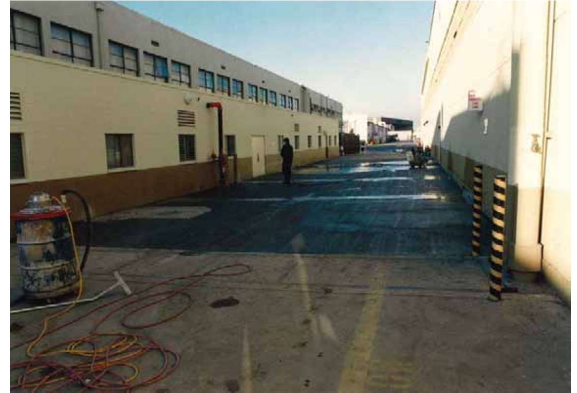
Building 102 - Contracts and Pricing Office, North Elevation, San Diego, California, date unknown. Teledyne-Ryan Archives.
