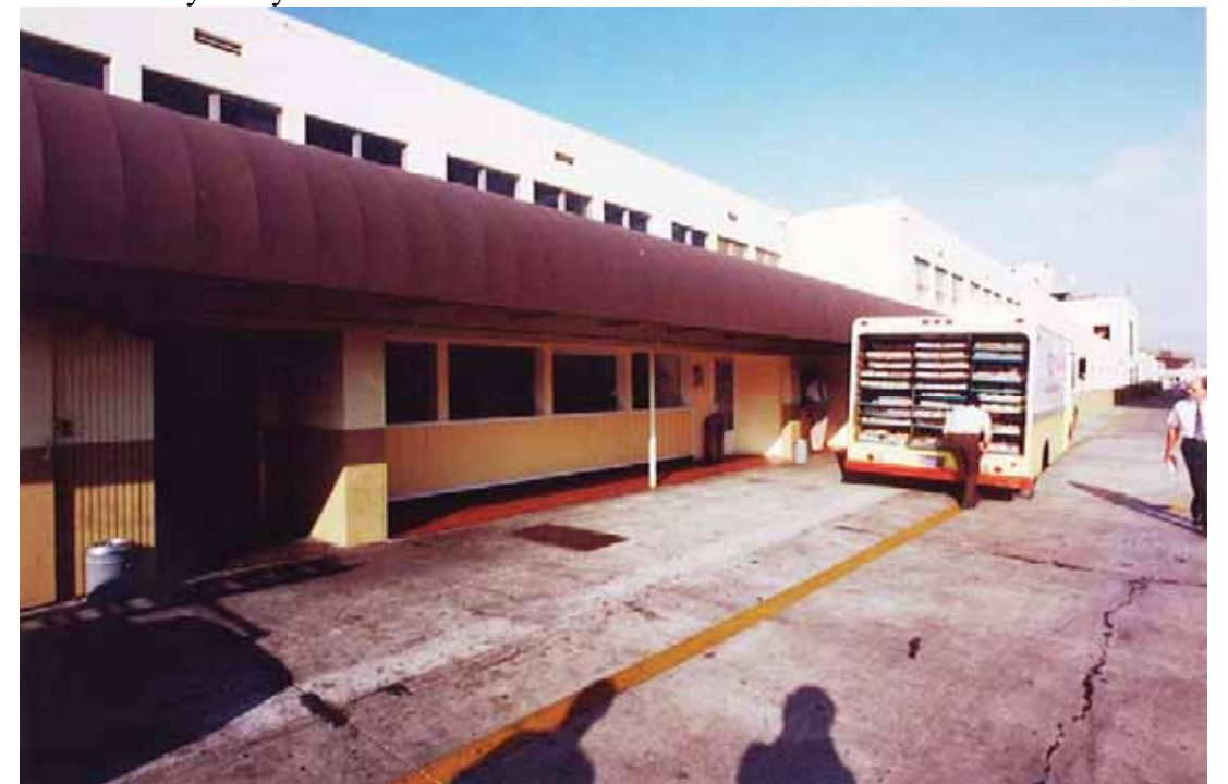
Building 102 - Contracts and Pricing Office, North Elevation, San Diego, California, date unknown. Teledyne-Ryan Archives.
