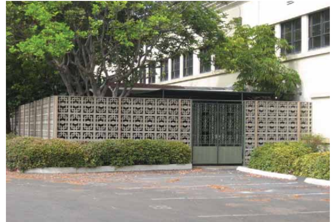
Building 102 - Contracts and Pricing Office, garden wall detail, facing Northwest, San Diego, California, October 2009.
