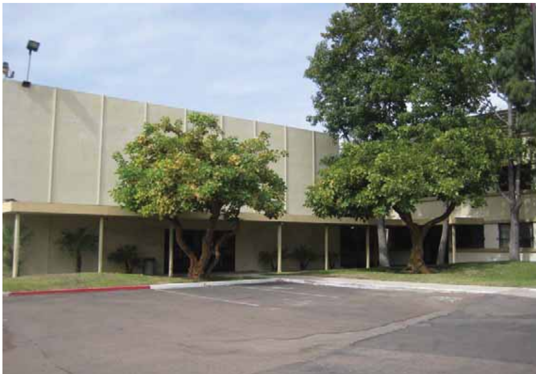
Building 102 - Contracts and Pricing Office, connection corner of Buildings 102 and 105, facing northwest, San Diego, California, October 2009.
