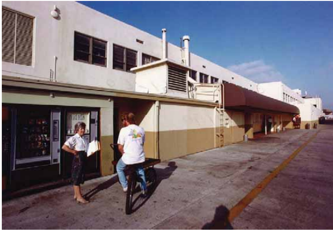
Building 102 - Contracts and Pricing Office, North Elevation, San Diego, California, date unknown. Teledyne-Ryan Archives.
