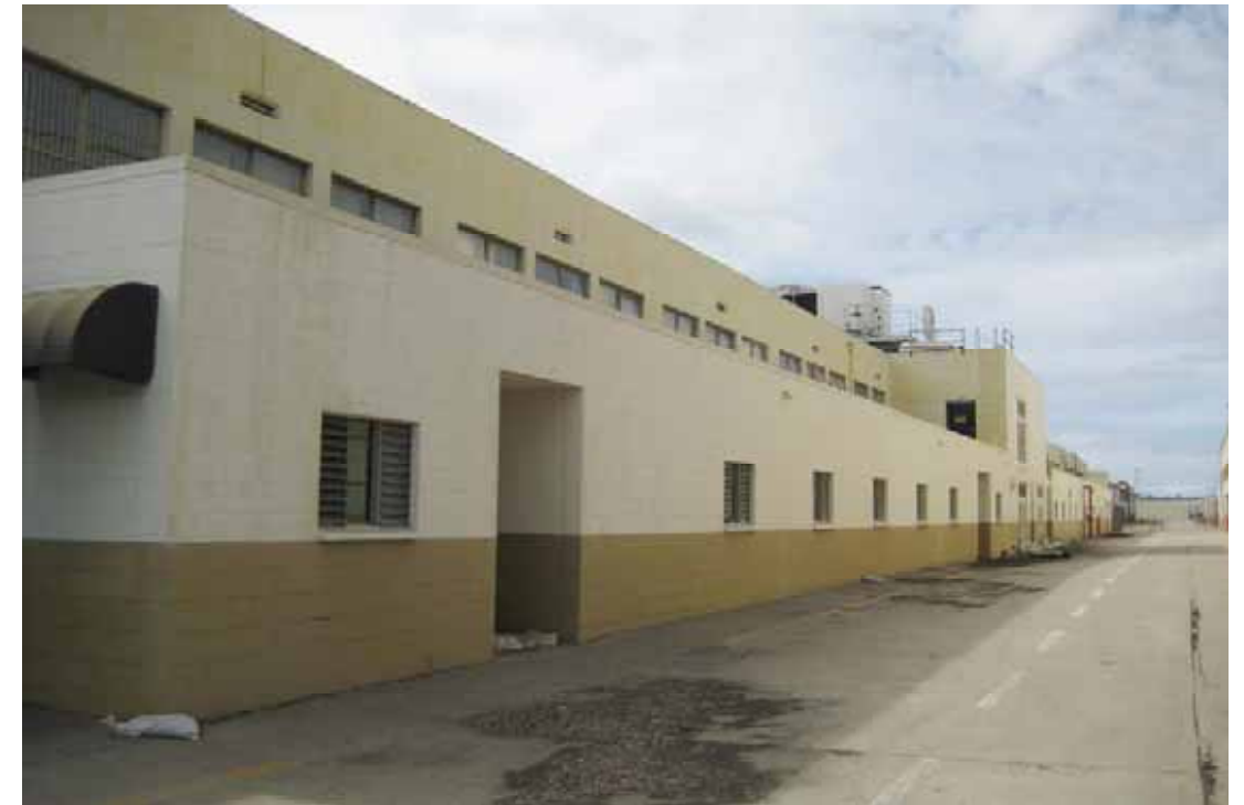
Building 102 - Contracts and Pricing Office, North Elevation, facing Southwest, San Diego, California, October 2009.
